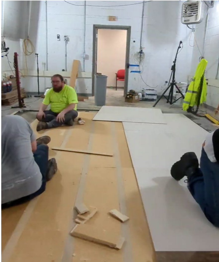
Photo No. 3 Construction of Test Specimen
